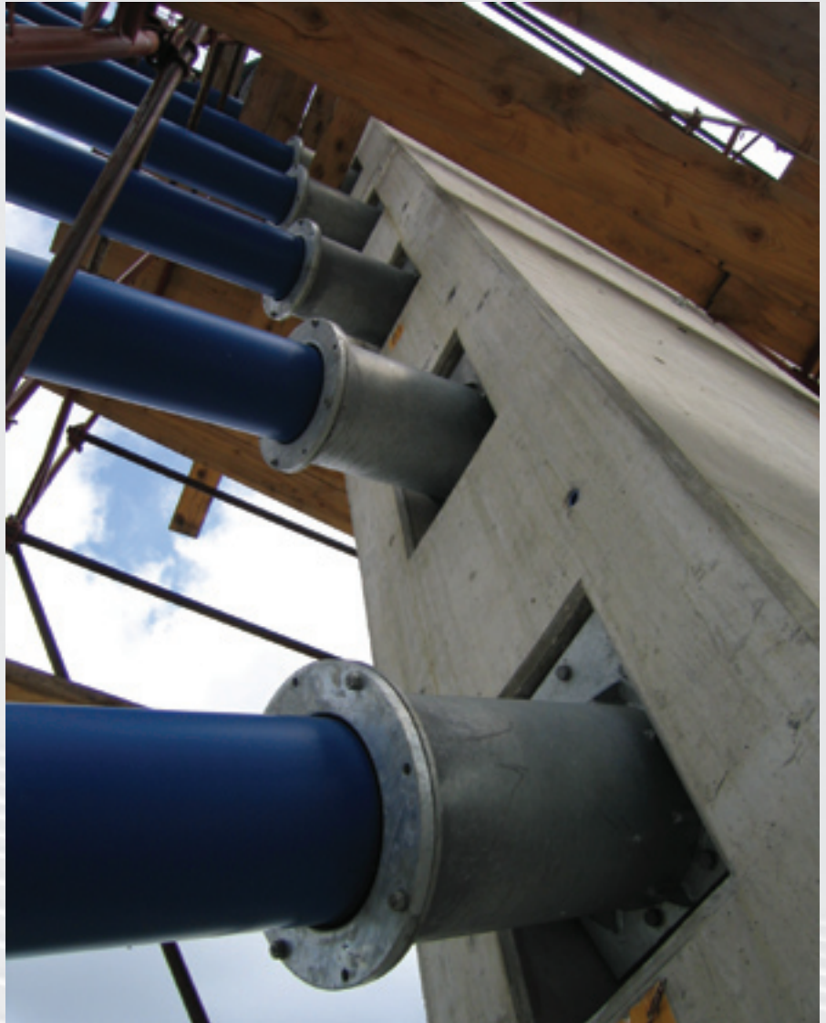
Installed Saddle Construction
