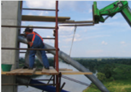
Saddle Pipe Installation
