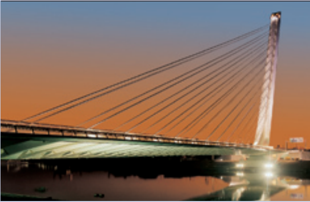
Alamillo Bridge, Sevilla, Spain 28 DYNA Bond® Stay Cables Maximum cable length: 292 m Cable size: DB-E61
