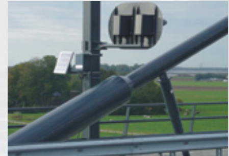
Installed External Damper
