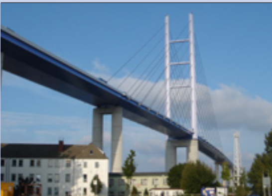
Ziegelgraben Bridge, Germany 32 DYNA Grip® Stay Cables Maximum cable length: 176 m Cable size: DG-P37
