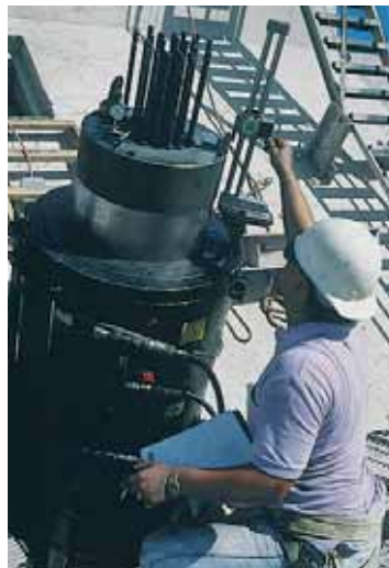
measurement of piston stroke
